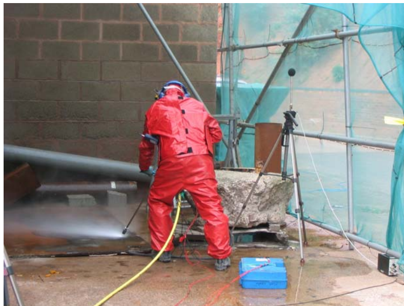
Figure 7 Water jetting towards workpiece at Site B
