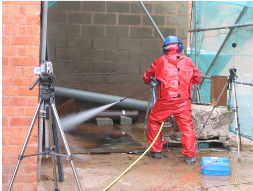
Figure 6 Free air water jetting at Site B
